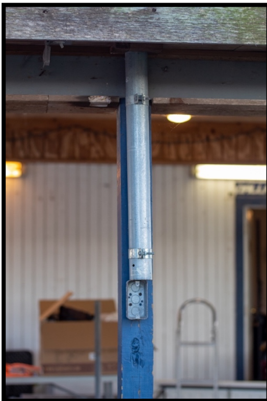
Photograph 42: The light pole is being held up by an empty electrical box. Its sole purpose is to support the pole.
