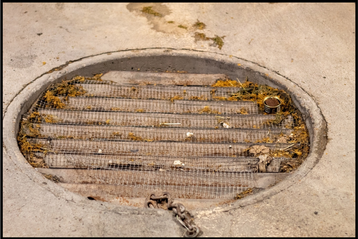
Photograph 92: George was tired of constantly having to unclog the drain, instead he put a wire mesh to stop the trash from going down.
