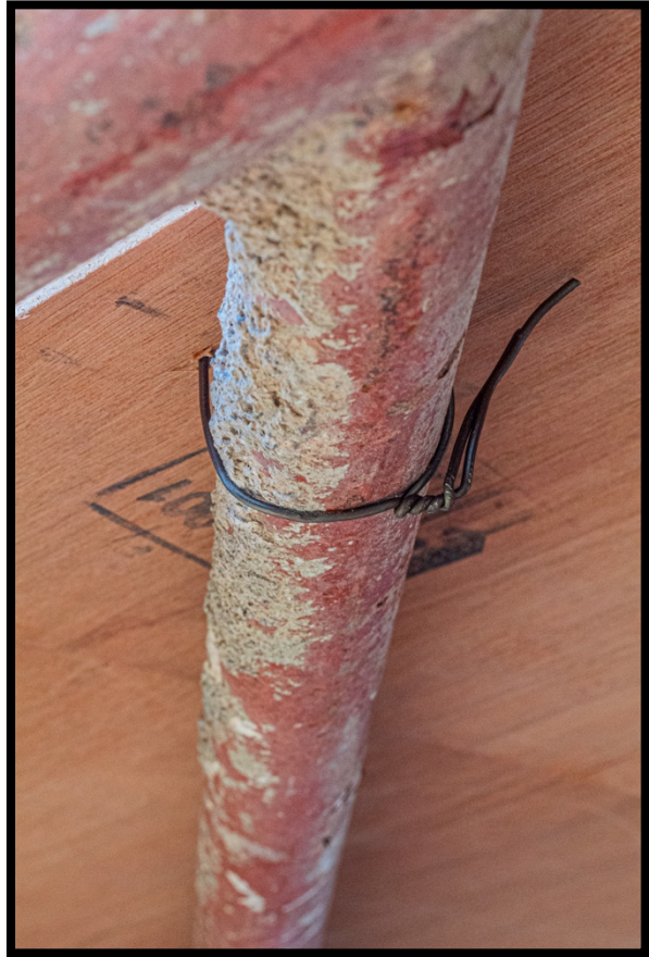
Photograph 60: The wood was held down to the frame of the ramp using what Jorge calls "Mexican zip ties", pieces of wire.
