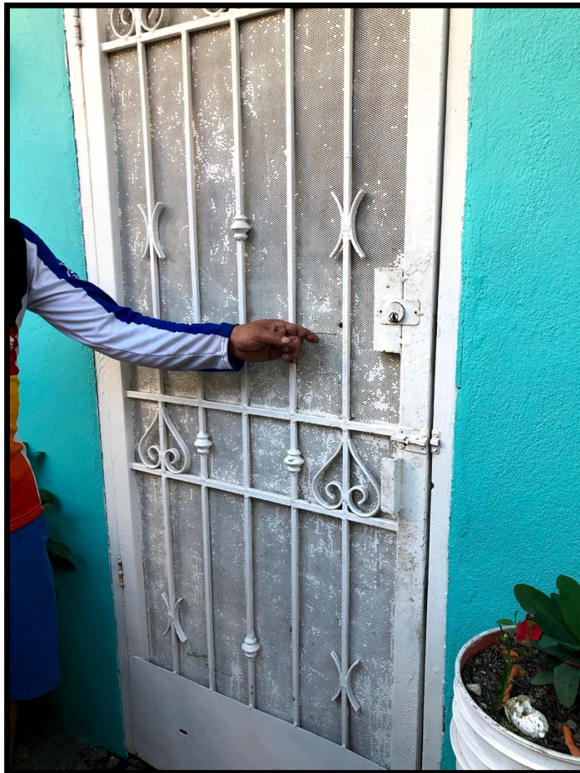
Photograph 141: This door could only be opened from the inside, to solve this my grandma made a whole in the mesh and attached a wire that can be pulled from the outside.
