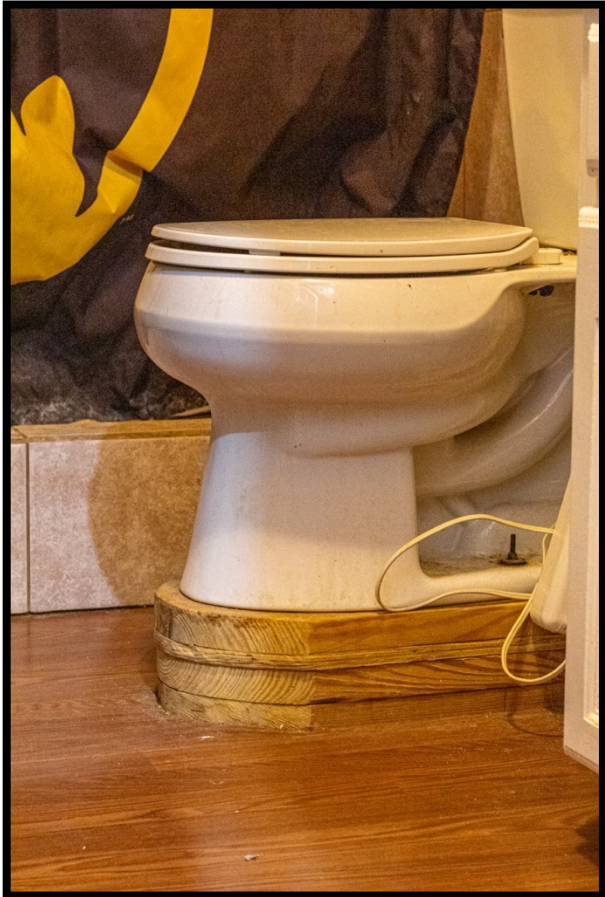
Photograph 49: When Jesse's elderly mother was going to visit him, he wanted to make her as comfortable as possible. He used left over wood to raise a normal toilet up. Reducing the distance she had to squat down, making it easier for her to use this.
