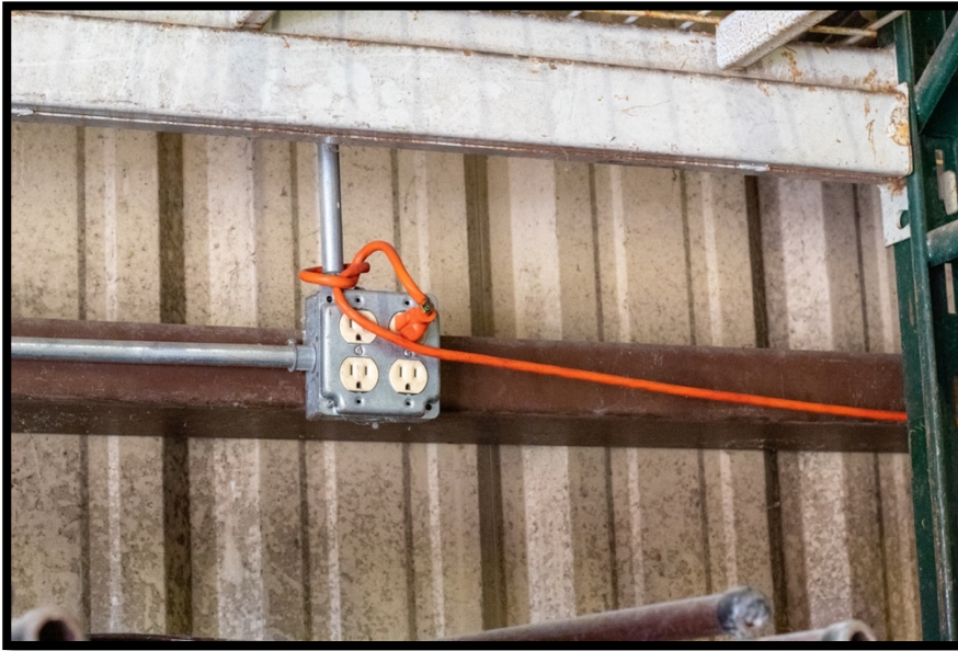
Photograph 138: This is how Felix plugs in his extension cords. Prevents it from being unplugged when it is pulled.
