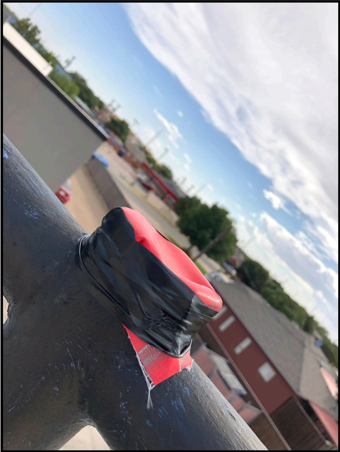
Photograph 145: A light post on the roof lost its cap, to prevent water from going into the pole and potentially touching wires we wrapped a piece of tarp around the whole with electrical tape.
