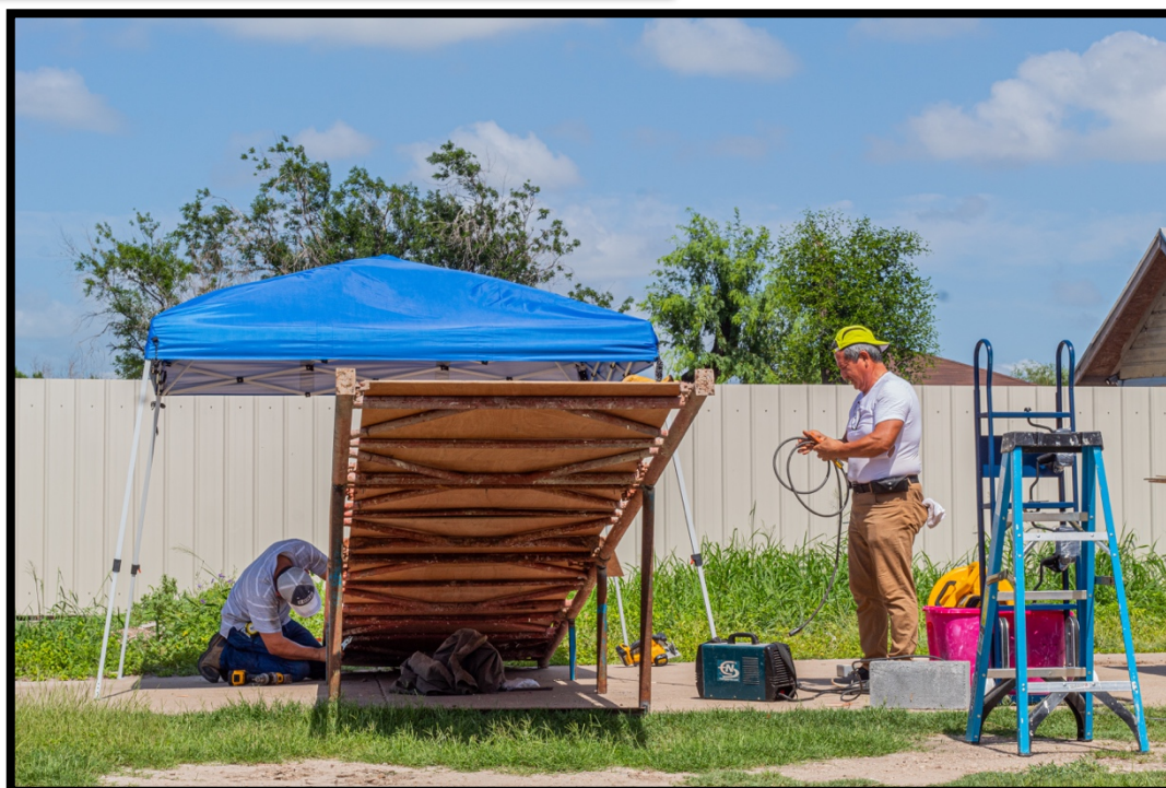
Photograph 57: Jorge Selvera, is doing the final touches on his biggest mexicanada yet. A ramp used to unload an 18-wheeler, made from recycled plywood and old scaffolds.
