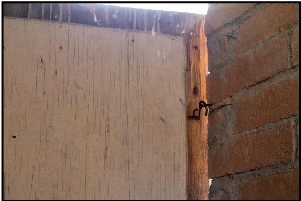
Photograph 119: Makeshift door hinge
