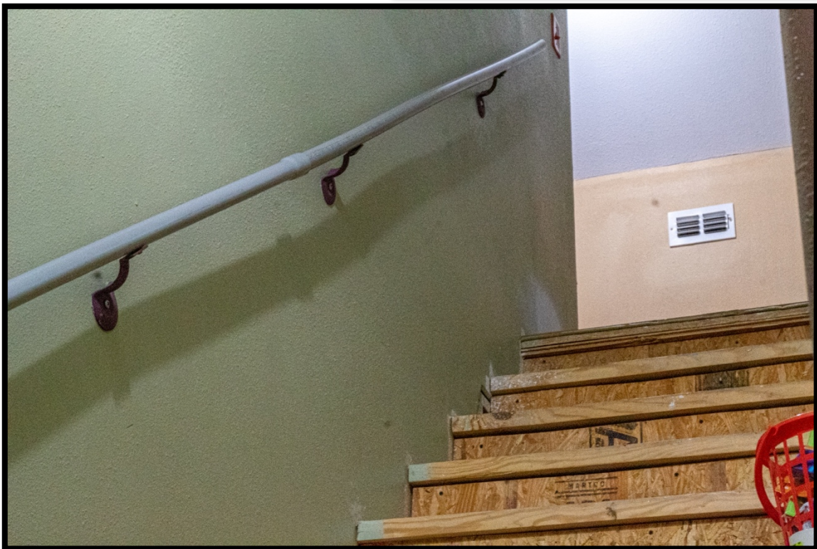
Photograph 50: Jesse also made a handrail on the stairs of his home for his mother, using PVC pipe.
