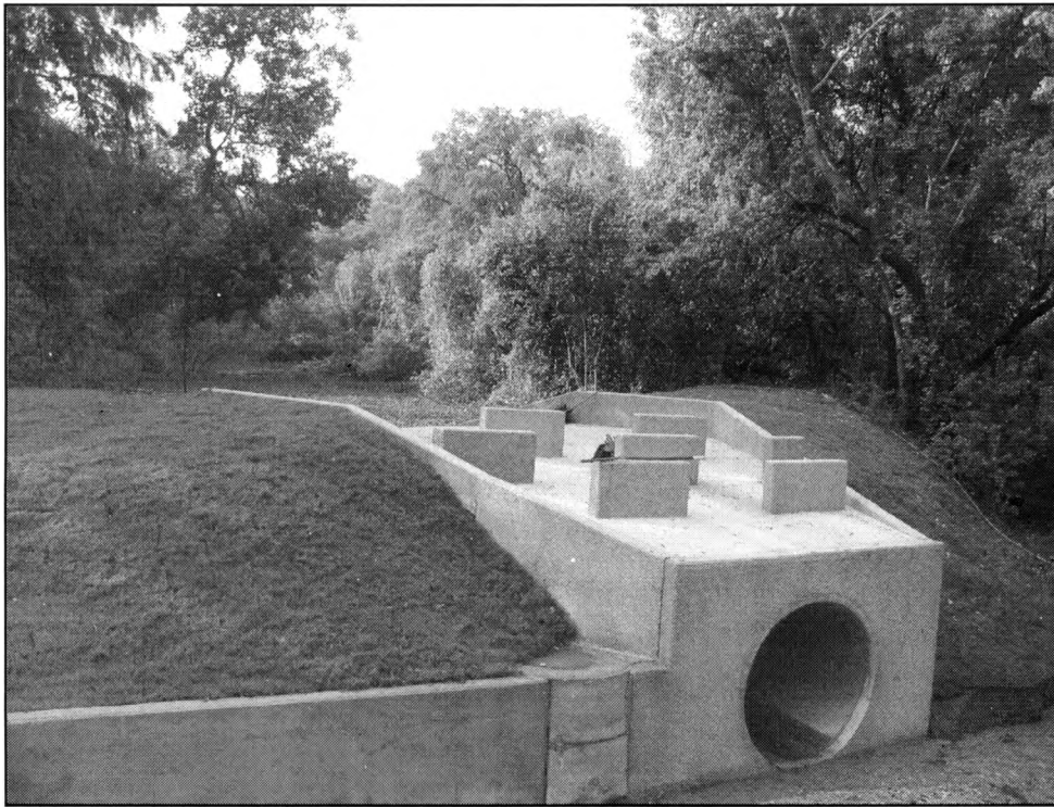
Figure 14. Installed flood control structure near Sessom Drive.
