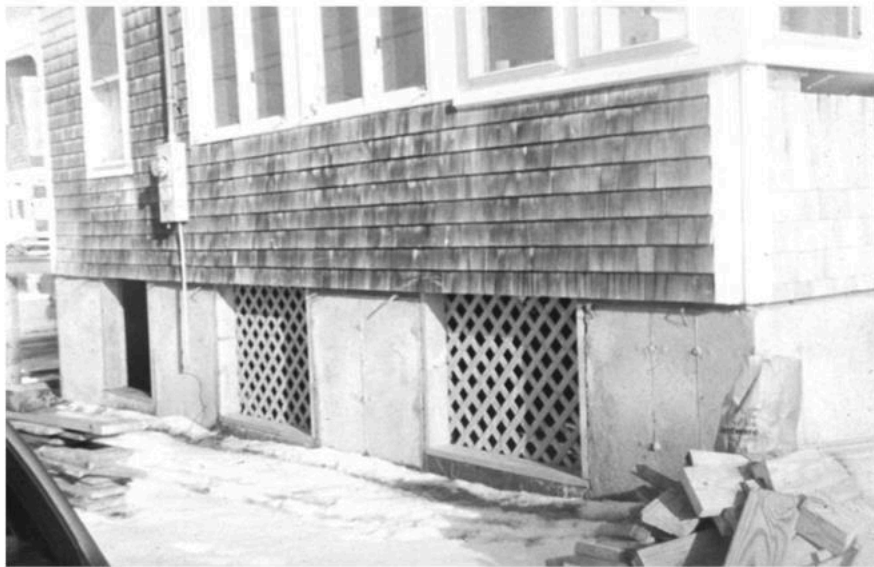
Figure 5-10: Building elevated on crawlspace with openings.
