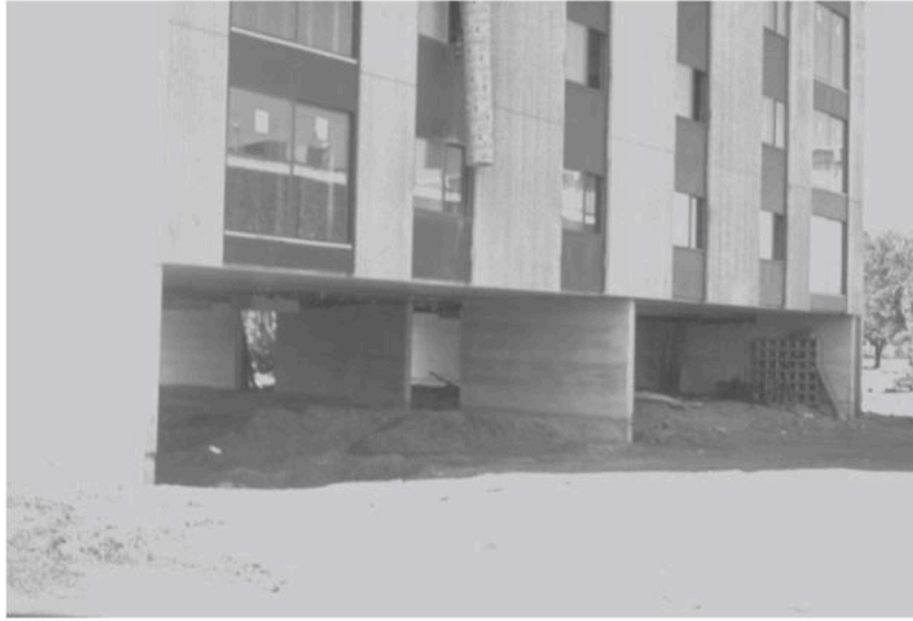
Figure 5-9: Building elevated on parallel stem walls.
