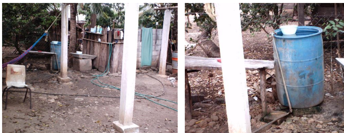
Figure 22. The wet area of a household with detail of the cistern (right) where hand washing and water retrieval is facilitated by the floating bowl. The pump for the piped water running throughout Babilonia Tercero is only run a few hours per day so cisterns are filled at this opportunity. The walled off area in the photo (left) contains a toilet fixture (one of the few in town – this is a prosperous household) and area for showering. Green hoses trail to the kitchen house for cooking and dish water.
