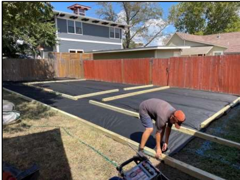
Figure 30. Laying the Landscape Timbers to Secure Weed Barrier Fabric and Create Boundaries.
