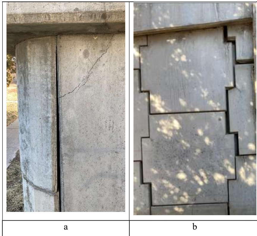
Figure 4-10 Wall issues a) panel bowing, b) misalignment of joints
