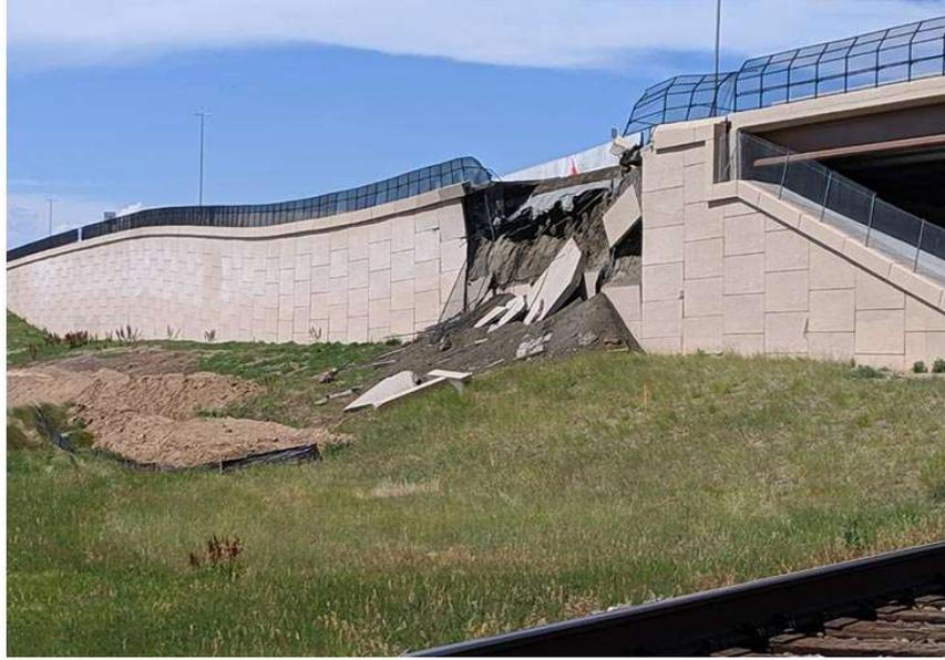
Figure 1-2 Colorado U.S. 36 Bridge MSE Wall Collapse (Shaw, 2019)
