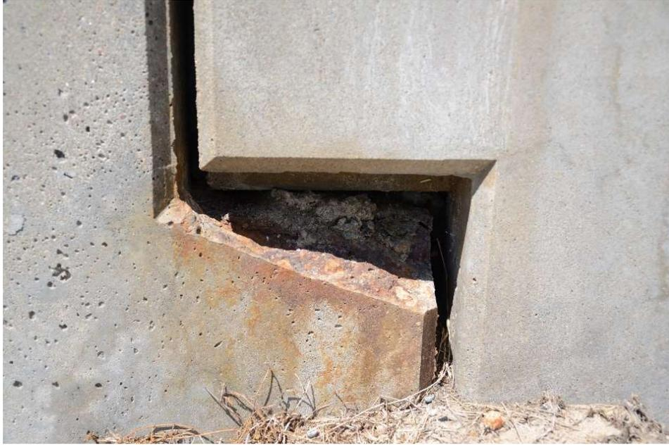
Figure 4-13 US-54 W to S Eisenhower Airport Pkwy Spalling
