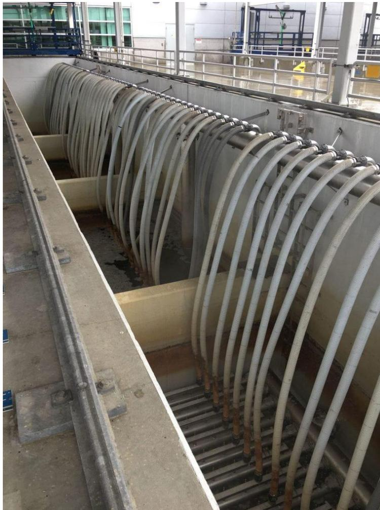
**Figure 2-2.** Microfiltration in OCWD GWRS (Photo courtesy of Dr. Keisuke Ikehata )
