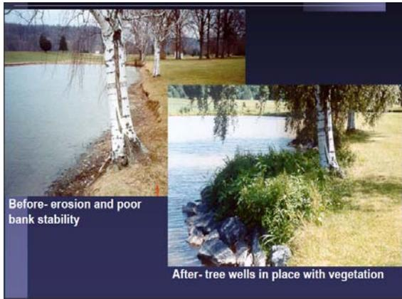
Figure 12 Bank erosion and runoff filter (Lampman
