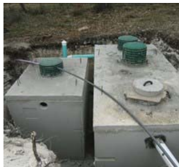
Figure 4. Biologically Accelerated Treatment plant during installation at research residence.
