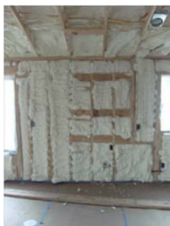
Figure 3. Open-cell spray foam insulation installed in the residence.
