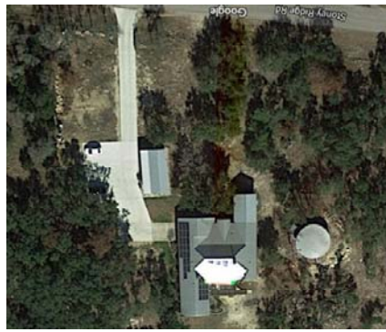
Figure 1. The residence as constructed.
