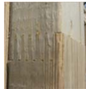
Figure 2. Finger-jointed stud used in the residence construction.
